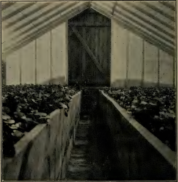
16.—Interior of twelve foot house, showing method of constructing south end and door.
